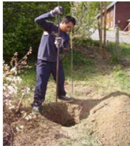
Figure 21: Site preparation, Ucwalmicw Centre Society
